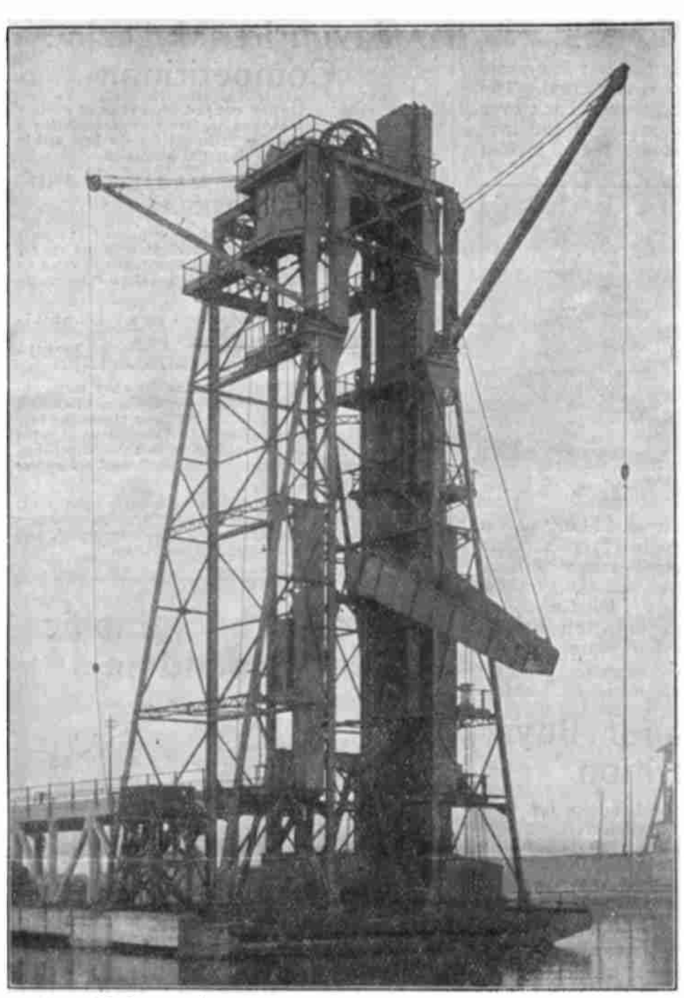
This Hydraulic Coal Hoist lifts a full truck of coals, weighing 30 tons, to a height of 60 ft.
